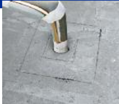
3) Place EternaPocket on roof and mark or scribe edge on roof surface as target for DoubleStick (MicroSealant Putty Tape).
