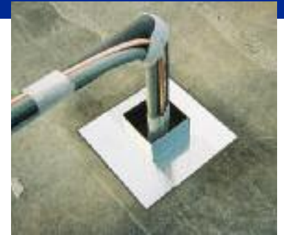
6) Apply pressure to activate MicroSealant adhesive. Go to Final Step #7.
