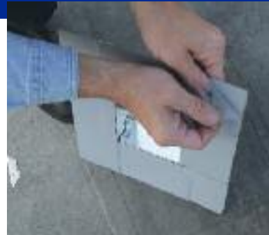
4) Apply TWO layers of DoubleStick (MicroSealant Putty Tape) to bottom of EternaPocket. *Be sure to remove BOTH release liners from each layer of tape. If doing Optional Step (below), allow tape to extend beyond the outer edge by 1/8".
