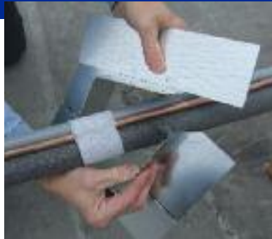
2) Fold EternaPocket around existing pipe or line.
