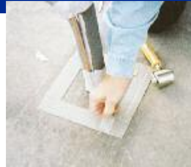
5) After removing top layer release liner, set EternaPocket in place. Use excess tape to fill in gap between pipe and roof before adding sealant.
