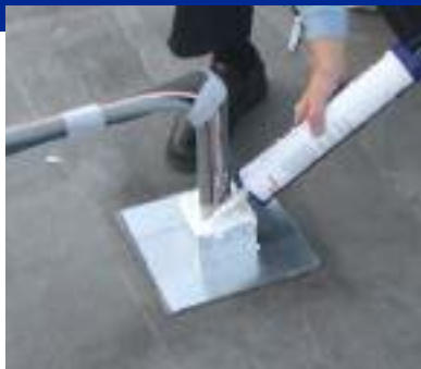
7) Fill EternaPocket with Sealant, using enough to create a "crown" of at least 1/4" above top edge of EternaPocket.
