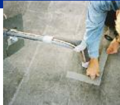
4) Clean surface with enclosed pad. Apply TWO layers of DoubleStick to roof surface. Be sure to remove BOTH release liners from each layer of tape. If doing Optional Step (below), allow tape to extend beyond the outer edge by 1/8".
