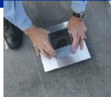
5) Clean surface with enclosed pad and set EternaPocket in place.
