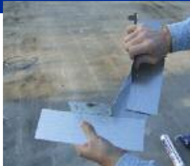
2) Fold EternaPocket into shape at hinges.
