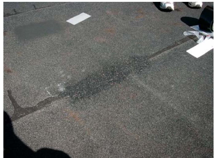
Figure 5: Roll or push granule into MicroSealant. Complete!
