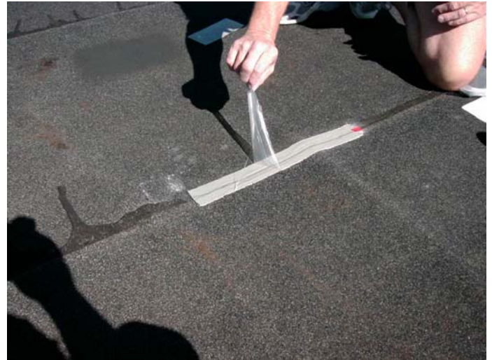
Figure 3: Remove 2nd release liner to expose top of MicroSealant surface.
