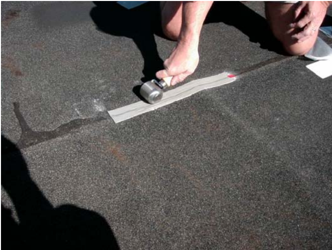
Figure 2: Roll or rub with pressure to activate wetting-in (fusing) action.
