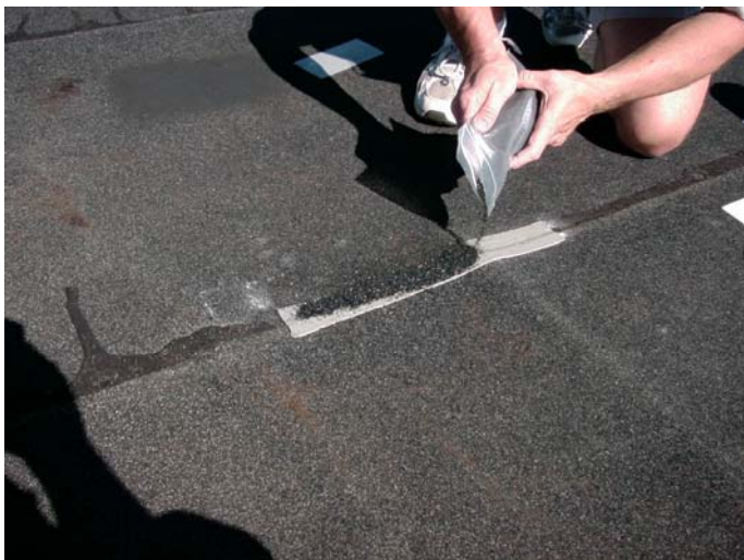
Figure 4: Pour matching granule onto exposed EternaBond MicroSealant. Matching granule can often be found in the gutters, etc.
