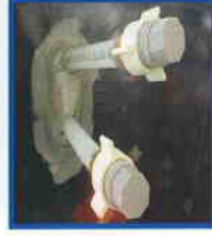
Fix Drain Pipes
