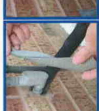
Remove liner, twist into rope and press into place. DONE!
