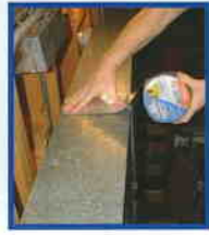
Indoor Ductwork Sealing
