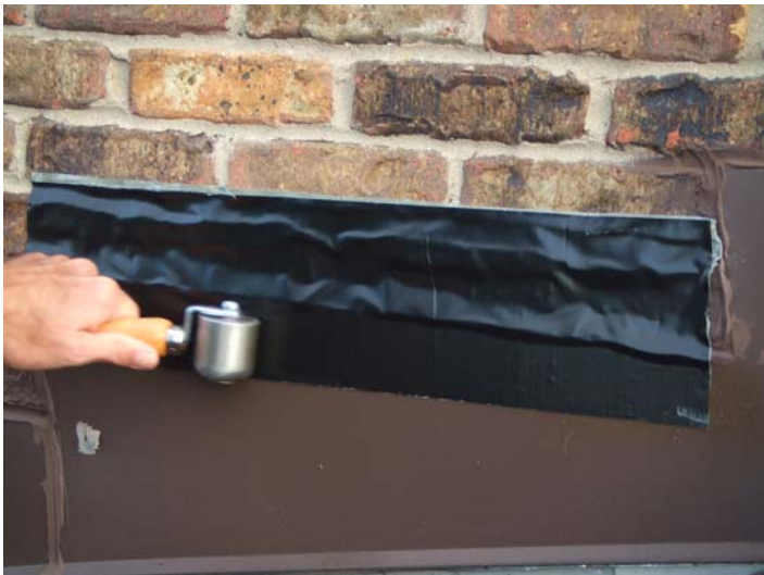
Figure 3: Roll or rub with pressure. Complete! By combining EternaBond DoubleStick and RoofSeal you have made an EternaBond MicroSealant tape with a custom profile to match the wall profile.
