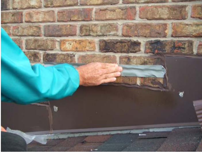
Figure 1: Apply EternaBond DoubleStick to wall in mortar joint. Remove 2nd (top) release film.
